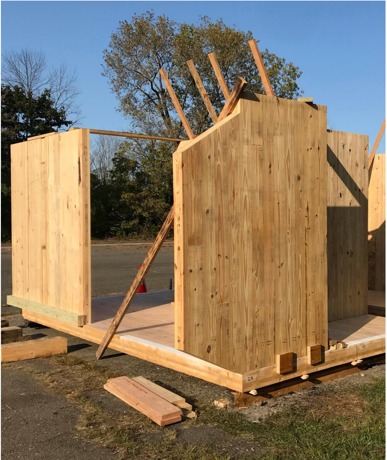
Fig. 20: Mass timber test assembly, Yale Regenerative Building Lab
